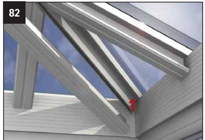
82 Complete the installation of 'T' shaped claddings by knocking on the Georgian claddings. Again, start at the ridge and work down to the eaves.
