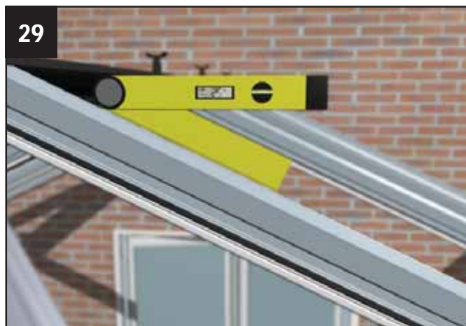
Check that the pitch of the roof is correct. Your Surveyor should have provided a drawing/a copy of the roof confirmation which displays the pitch.
