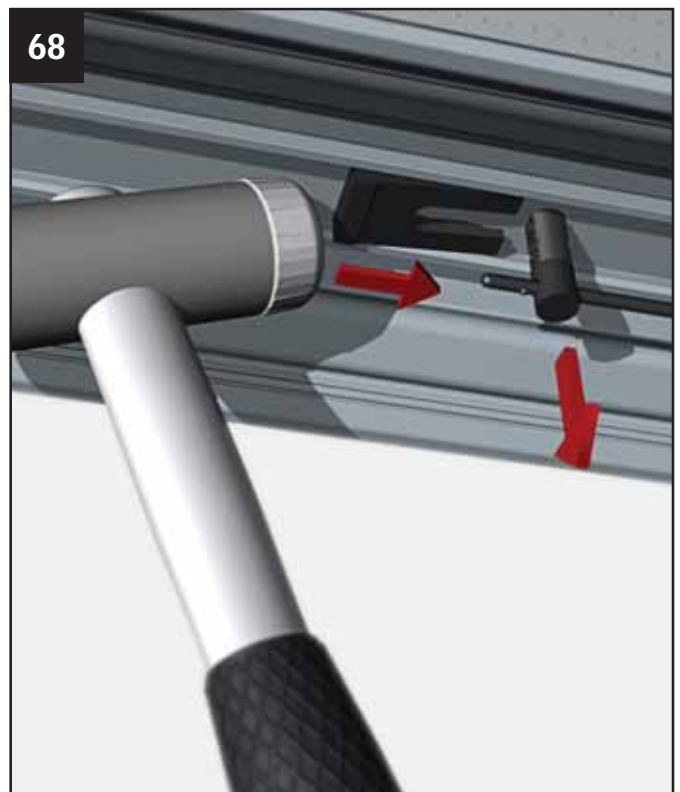
68 Pull down on the T bolt and tap the fixing wedge into place to secure the T bolt. Cut off the excess T bolt below the fixing wedge.
