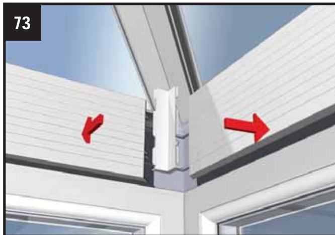
73 Slot each section of internal fascia into the corner jointer and tap the fascia onto the barbs of the eaves beam. Fit Ultraselect strips into the slots in the fascia
