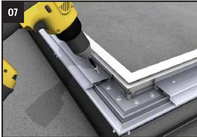
Using the fixings provided, attach the lantern undercarriage, 50mm from the back edge and at 500mm ctrs.
