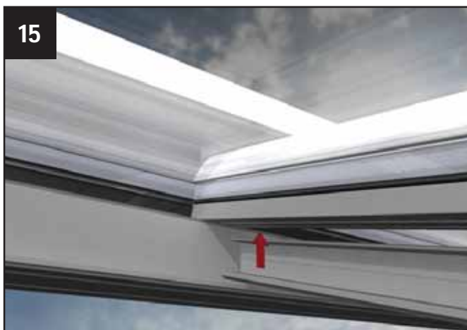
Clip on the 'T' shaped claddings.
