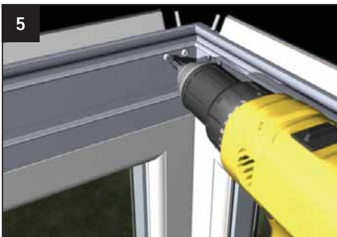
5 Securely fit the two M5 x 12mm tapite screws.
