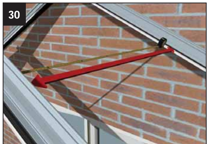
Check that the starter bar and first transom bars are parallel.
