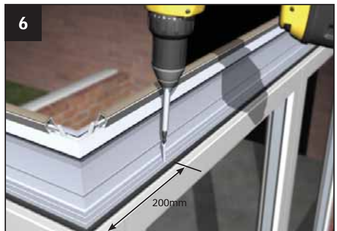
6 Securely fit the eaves beam to the frames using for example, 38mm x 4.8mm screws in the position shown. Fix down at 450 centres and within 200mm of each corner. For 60mm frames use the inner eaves extrusion line and outer line for 70mm frames. Always screw down. (Not supplied)
