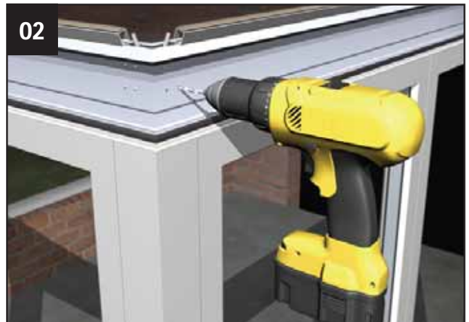
02 Two pilot holes already exist in the next piece of eaves beam – drill two more at 4.5mm diameter through the eaves beam and the cleat and then securely fit the four M5 x 12mm tapitpe screws.
