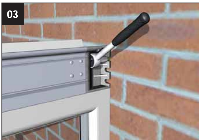
03 Where the eaves beam sits against the host masonry wall, it has a structural moulding attached to the eaves beam. This has three fixing positions cast into it to allow attachment into masonry – choose the hole that directly lines up with solid masonry and drill a 10mm hole into the host wall. Attach the structural moulding using the M8x80mm anchor supplied. Silicone seal the gap where the moulding attaches to the eaves beam.
