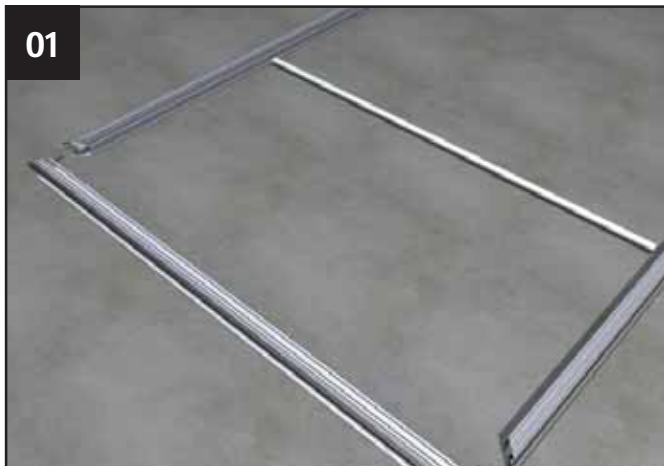
01 Layout the pieces of the lantern eaves beam.
