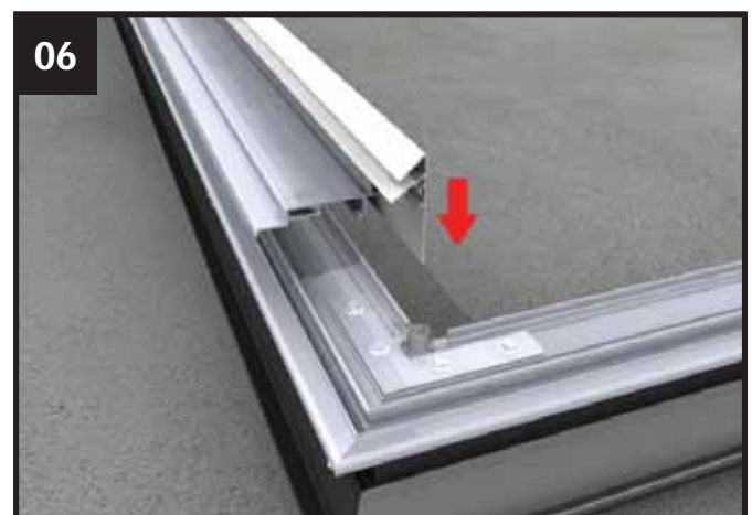
06 Lay the lantern undercarriage (aluminium and PVC sections) in position.
