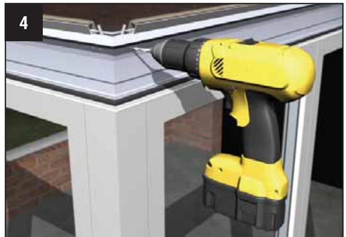
4 Using the pre-drilled pilot holes, drill two 4.5mm holes through the corner cleats.
