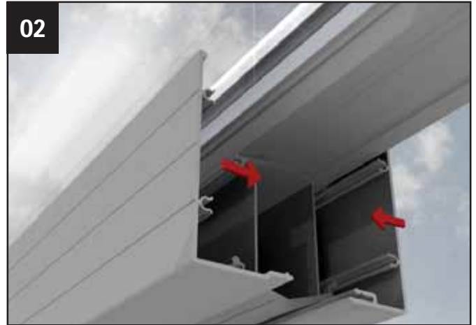
02 Take the two part cladding, attach each piece carefully to the aluminium bolster profile and 'zip' together.
