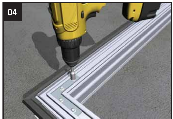
04 Fasten both fixings in both cleats on every corner
