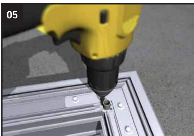
05 If supplied, fasten to each corner the tie bar drop rod fixing bracket to the underside of the lantern eaves beam.
